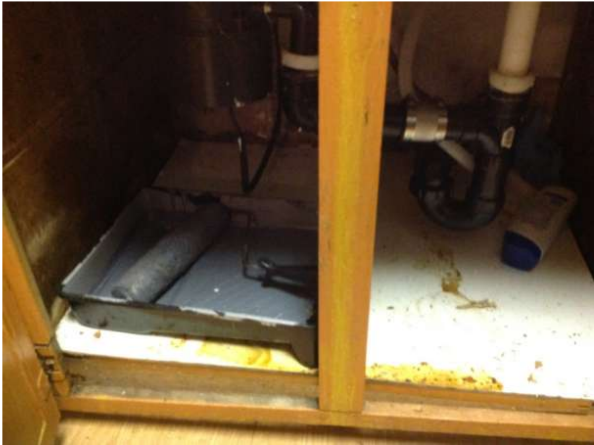
Image # 2: Under counter in the kitchen
