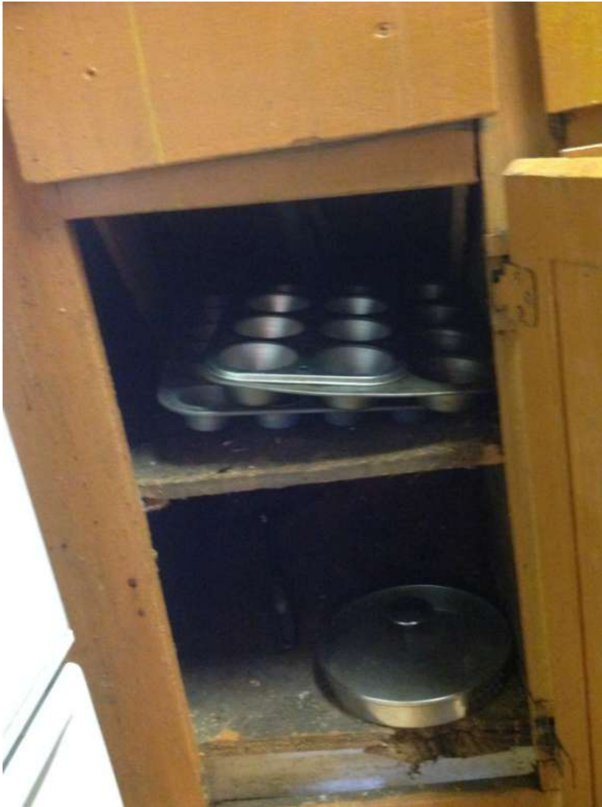
Image #4: Under counter in kitchen
