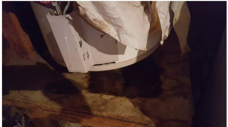
Figure 7: Paint Cans & Wet Area Under Hot Water Heater
